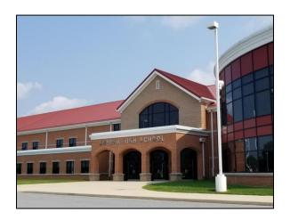
Similar to the adjacent Middle School, the exterior envelope is brick and split-face masonry in varying colors, with some areas of ribbed metal wall panels at upper areas. Masonry is in fundamentally good condition throughout. Large aluminum storefront / curtainwall, windows, and exterior doors are in generally good condition throughout, and include insulated glazing.
