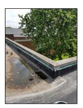
additional interior water damage. As part of this program, remaining cast stone copings should be covered with new prefinished aluminum copings to improve water integrity of the roof / exterior wall connection.
