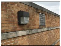
weathering of mortar joints has occurred, particularly around stone copings and windowsills. Walls show evidence of chronic wetness around downspout and overflow locations. A program of masonry cleaning and repointing in the mid-term future will help preserve strength and appearance.
