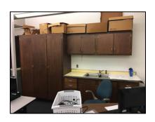
fixtures are well past their expected life span, show substantial wear and damage, and are not accessible. Casework in remaining unrenovated rooms should be replaced with new suite of fixtures to match renovated areas.
