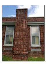
preserve strength and appearance. One item requires priority attention: an existing chimney on the east of B wing shows significant cracking. At a minimum, the cracks require repair and repointing. This chimney is believed to be abandoned and could be demolished to eliminate future problems.
