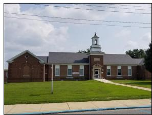
Structural systems and roof types vary by location, with mostly pitched roofs and some low-slope areas. Most pitched roofs have been shingled with a long-life synthetic slate material. Some low slope roof areas will require replacement in the near future.
