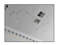
infiltration or leaks in acoustical panel or other ceilings. These must be investigated by District personnel, the water sources corrected as required, and damaged materials replaced.
