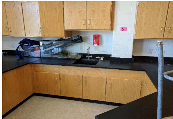
Photo #18 Typical Classroom Sink
