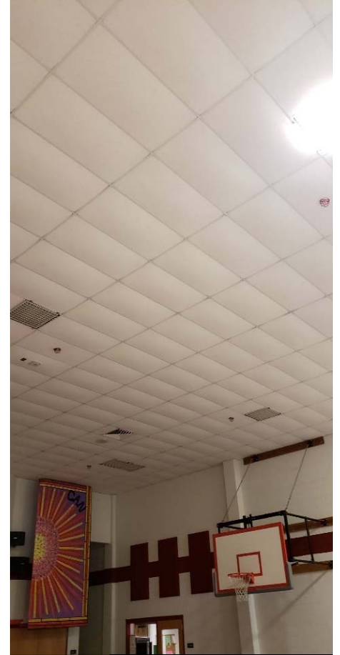
Photo #7 Lights and Ceiling in Gym/Auditorium/Cafe
