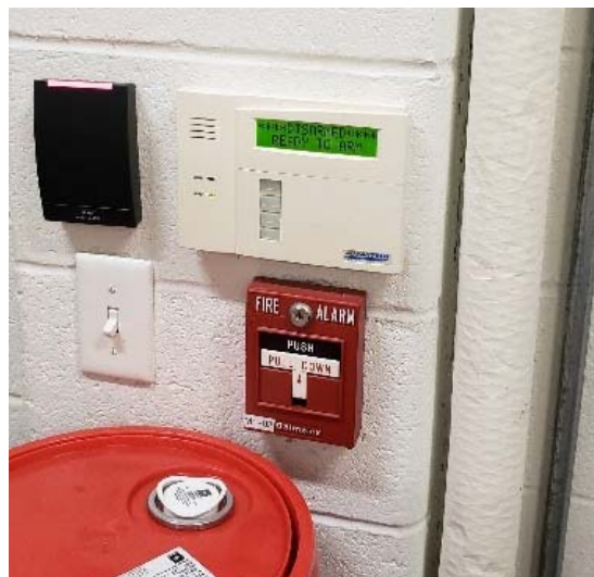
Photo #16 Typical Security Keypad and Card Reader
