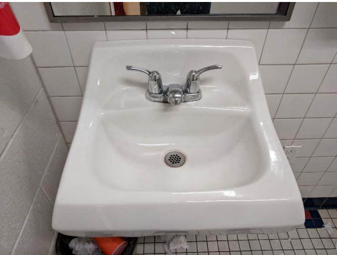
Photo #7 Typical Bathroom Lavatory
